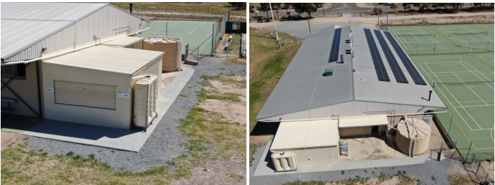
Lock Sports Centre—Kitchen Upgrade and Solar Installation
