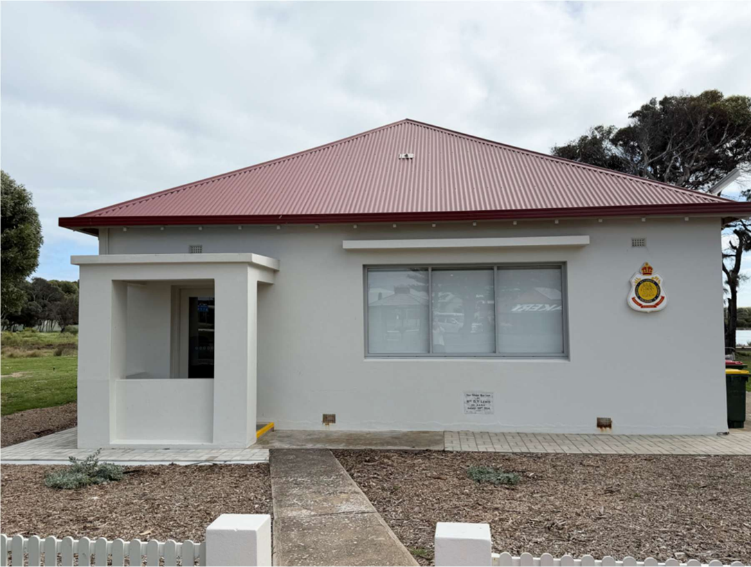
Front of Building
