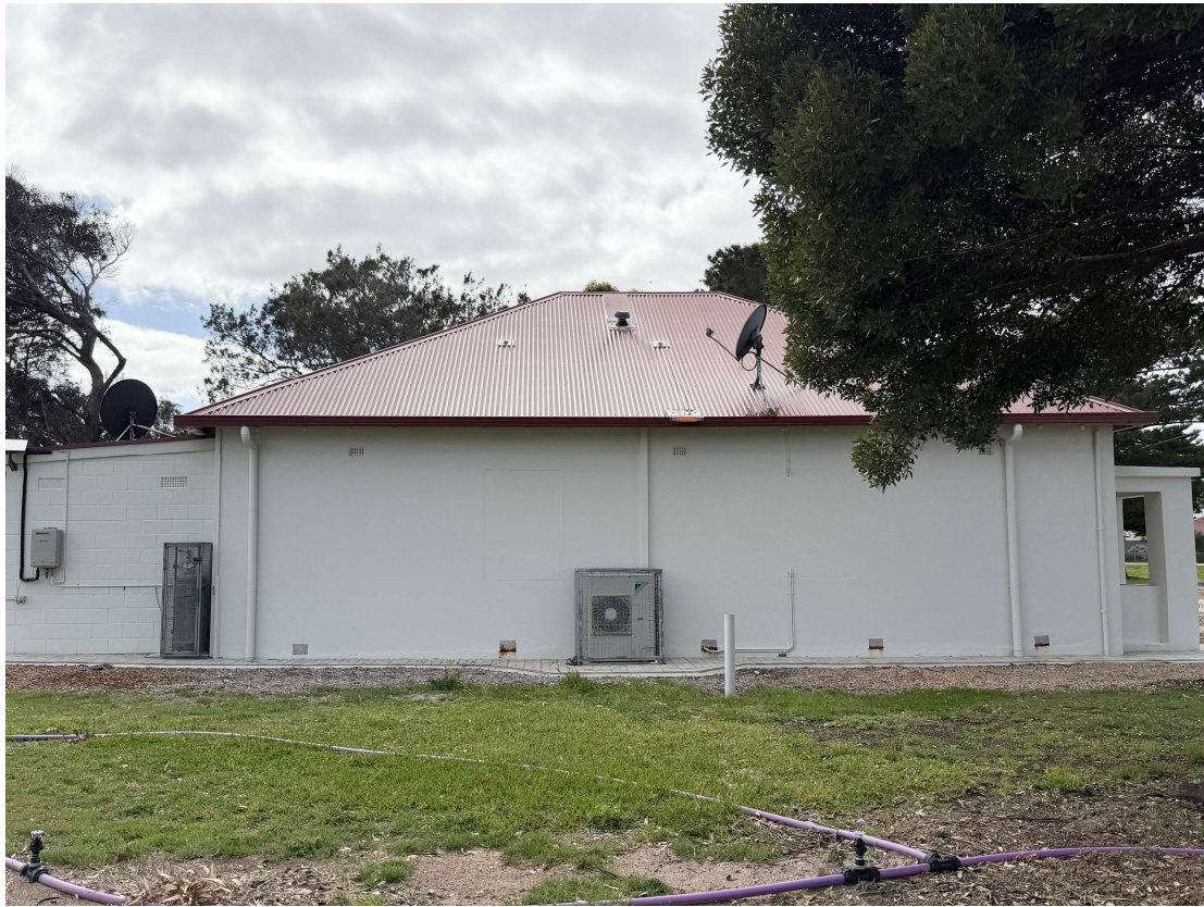
Side of Building
