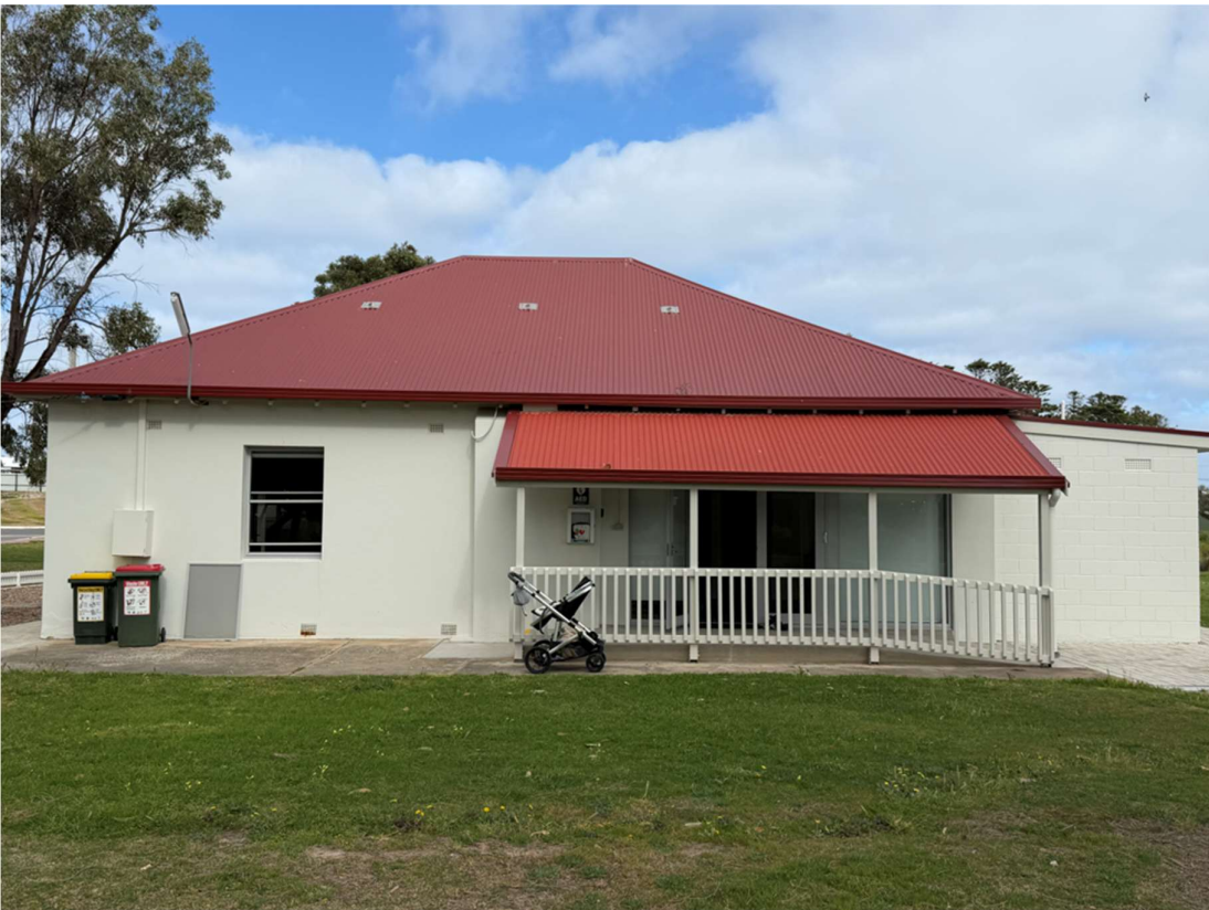
Side of Building
